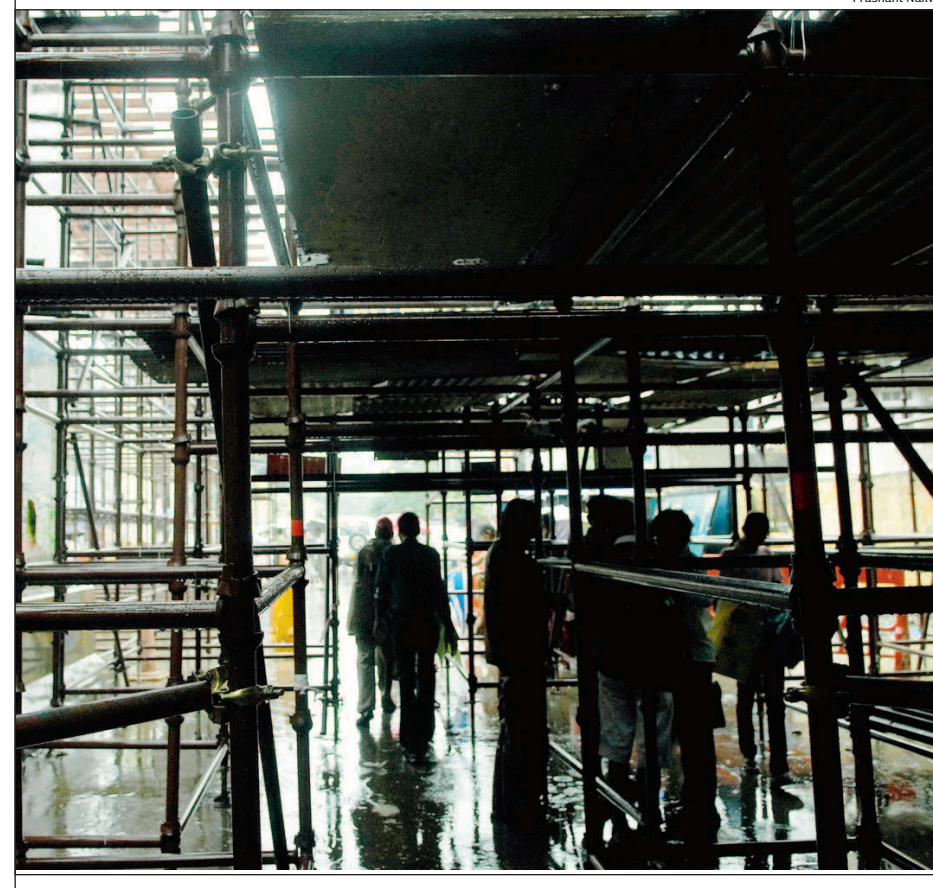
WORK IN PROGRESS: Work in full swing to connect the Metro corridor to the central railway and the skywalk near Ghatkopar station
